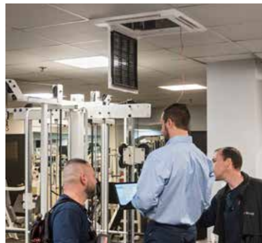
Chris Renna, center, connects the service tool to a compact cassette to ensure everything is operating correctly.
