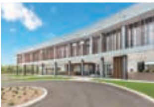
Fujitsu General (Aust.) Pty Ltd. (Australia)
