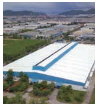
Fujitsu General (Thailand) Co., Ltd. (Thailand) FACTORY-2
