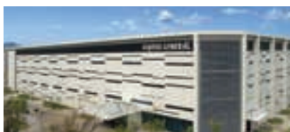
Fujitsu General Air Conditioning R&D (Thailand) Co., Ltd. (Thailand)
