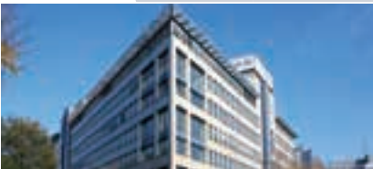
R&D Center in Fujitsu General (EURO) GmbH (Germany)
