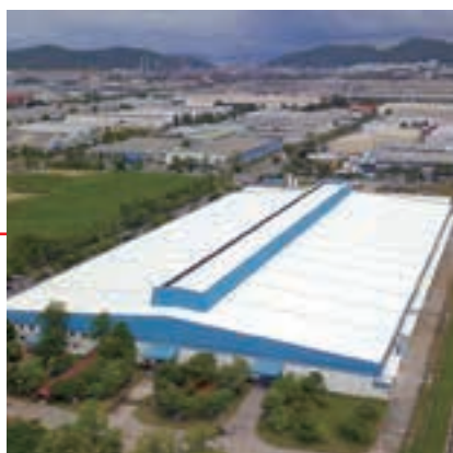
Fujitsu General (Thailand) Co., Ltd. (Thailand) FACTORY-2
