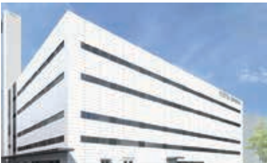
Technology Research Building (Japan)
