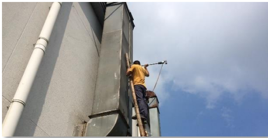
Duct inspection at Fujitsu General Central Air-conditioner (WUXI) Co., Ltd.
