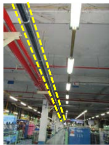
After updating (inside dotted line: polyethylene pipe)
