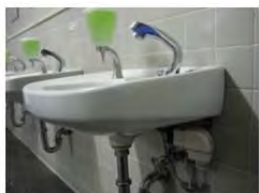
Renovated water flush at head office
